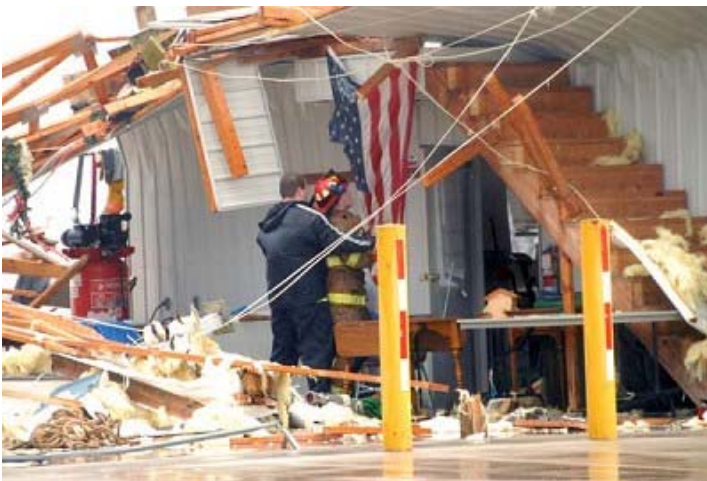
Trimble County— Milton Fire and Rescue Station 2
