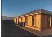
18 EXISTING CONDITIONS SCALE: NA
