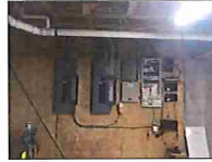
14 EXISTING CONDITIONS SCALE: NA
