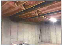
11 EXISTING CONDITIONS SCALE: NA
