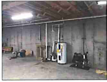
6 EXISTING CONDITIONS SCALE: NA
