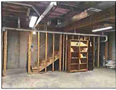
1 EXISTING CONDITIONS SCALE: NA
