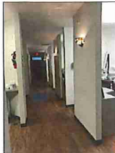
7 EXISTING CONDITIONS SCALE: NA
