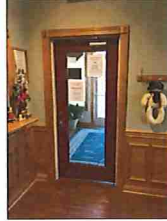
15 EXISTING CONDITIONS SCALE: NA
