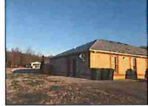
19 EXISTING CONDITIONS SCALE: NA
