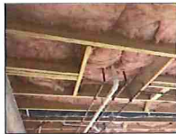
12 EXISTING CONDITIONS SCALE: NA
