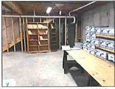
3 EXISTING CONDITIONS SCALE: NA
