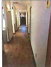
8 EXISTING CONDITIONS SCALE: NA
