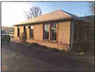
17 EXISTING CONDITIONS SCALE: NA
