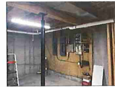
3 EXISTING CONDITIONS SCALE: NA
