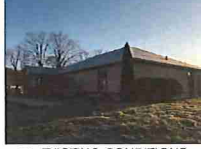
20 EXISTING CONDITIONS SCALE: NA
