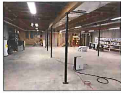
2 EXISTING CONDITIONS SCALE: NA
